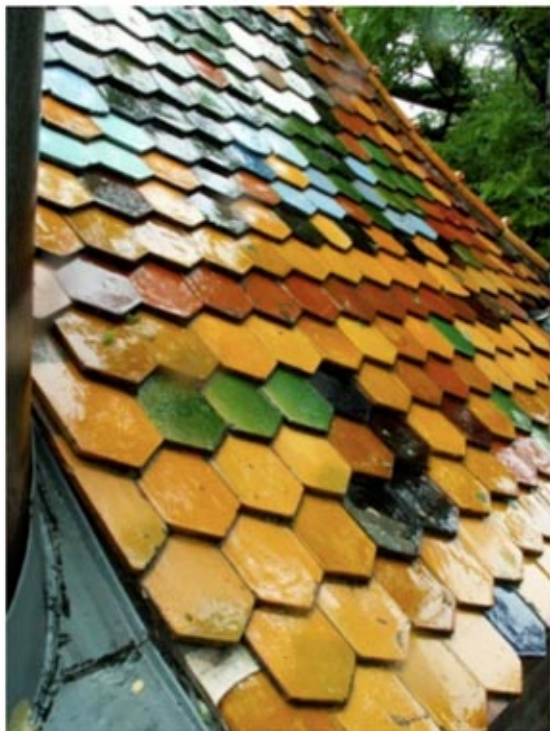
Zsolnay tiles on the roof of an old building at the factory
