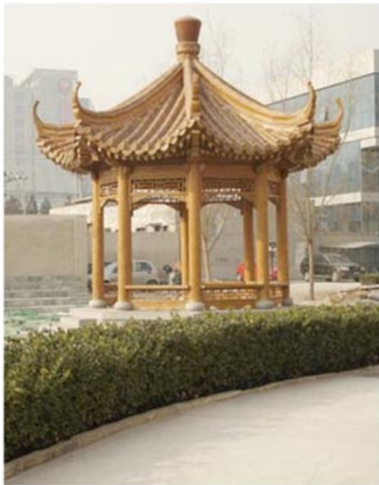
Glazed tiles pavillion
